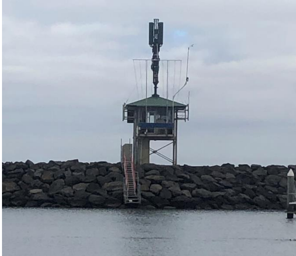
Start Tower 2020. Scaffold stairs boat access – Monthly inspection by Scaffold Solutions.
