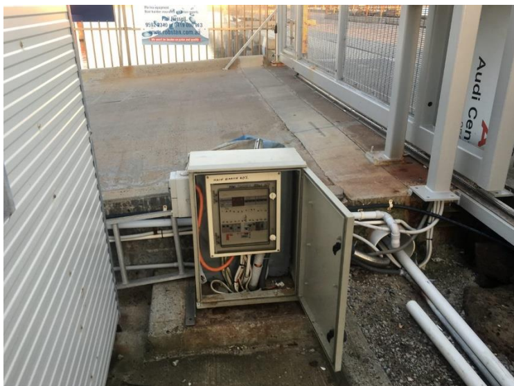
Electrical Shut-Off – Brighton Pier
